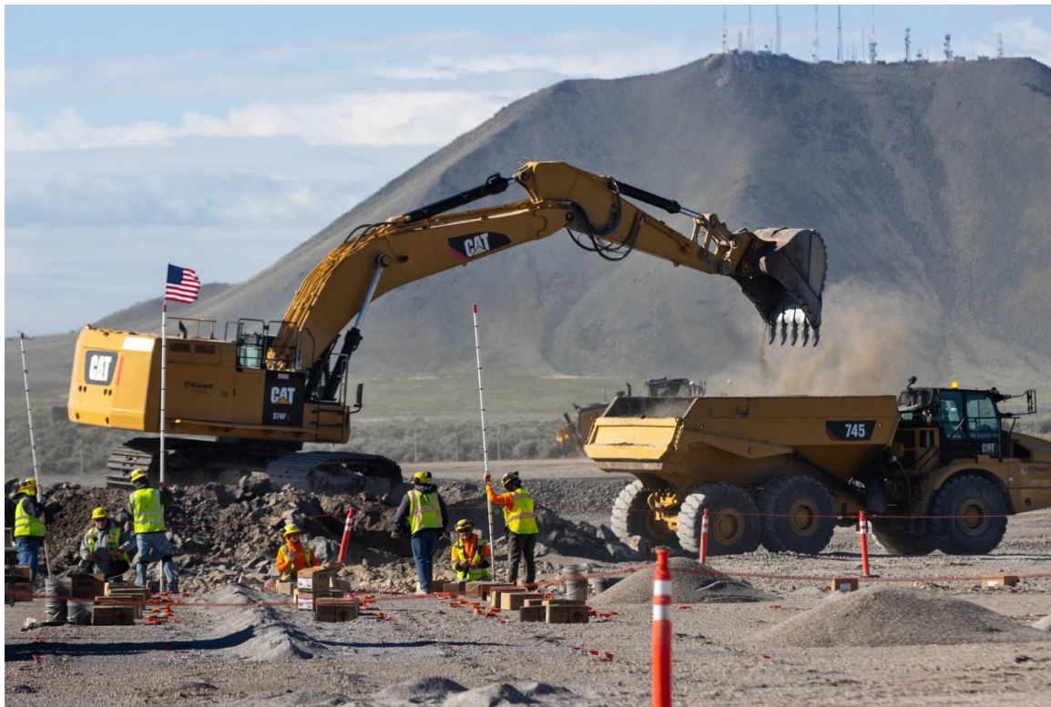
Construction takes place at the Aurora Powerhouse, an Oklo reactor site at Idaho National Laboratory.
