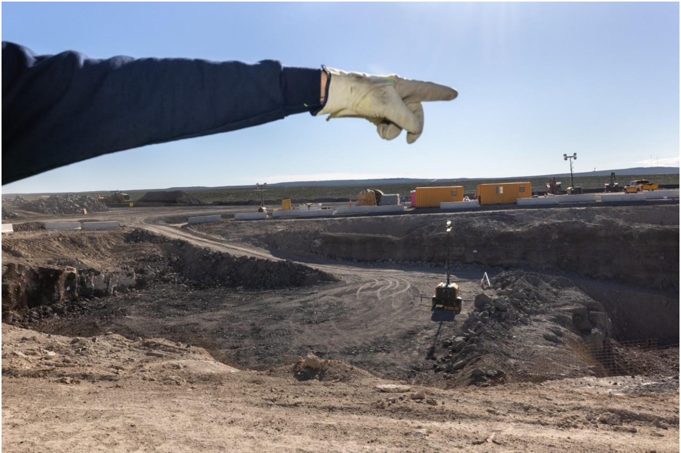
Construction at the Aurora Powerhouse, an Oklo reactor at Idaho National Laboratory.
